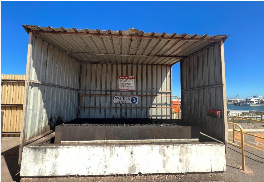
Left – Bunded Waste Oil Receptacles (Fishing Boat Harbour)
