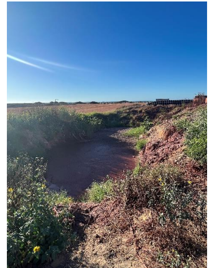
Sump Behind Bunkers 1 and 2
