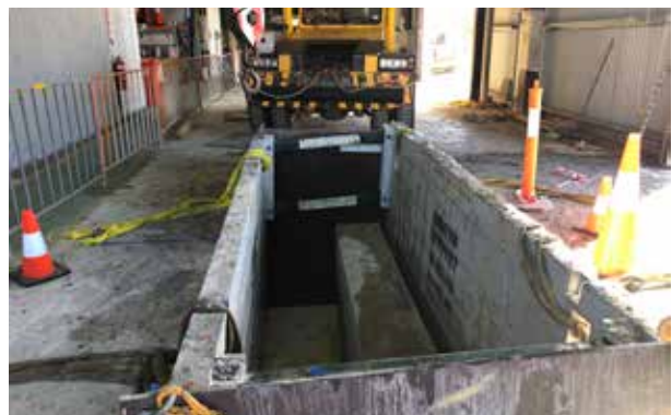
Dead-man & Tieback installation – Inside of workshop
