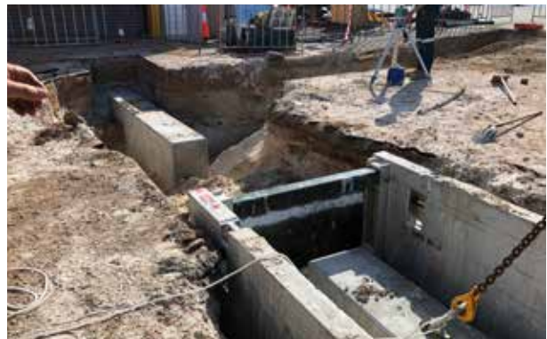
Dead-man & Tieback installation – outside of workshop
