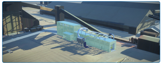
New $52 million Truck Unloader includes an enclosed design which incorporates dust extraction
